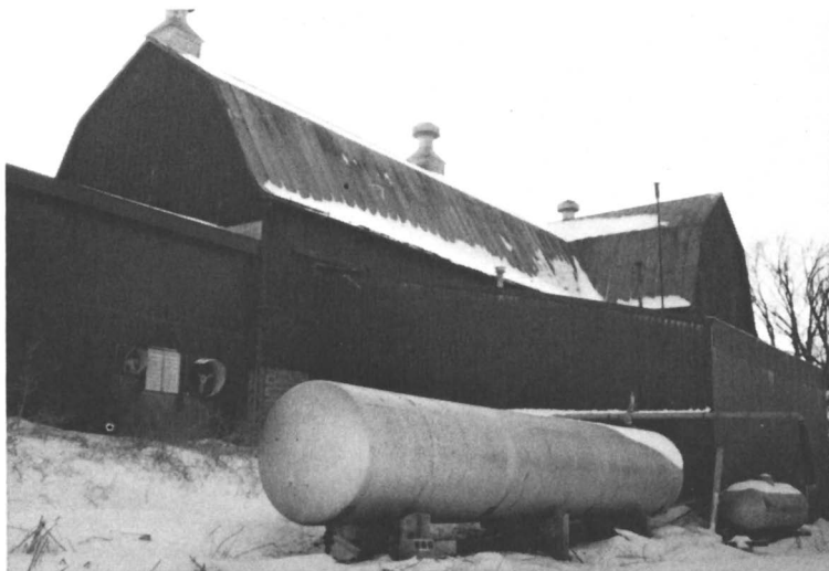
Figure 2. A 16,000 poultry layer operation in a converted dairy barn with an anaerobic-digestion biogas plant in the attached shed in the foreground (W. Gibbons' farm at Ripon, Wisconsin)
